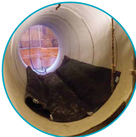
Placing – pillow plug should be positioned horizontally
