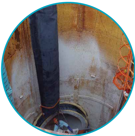
Inserting a folded pillow plug
